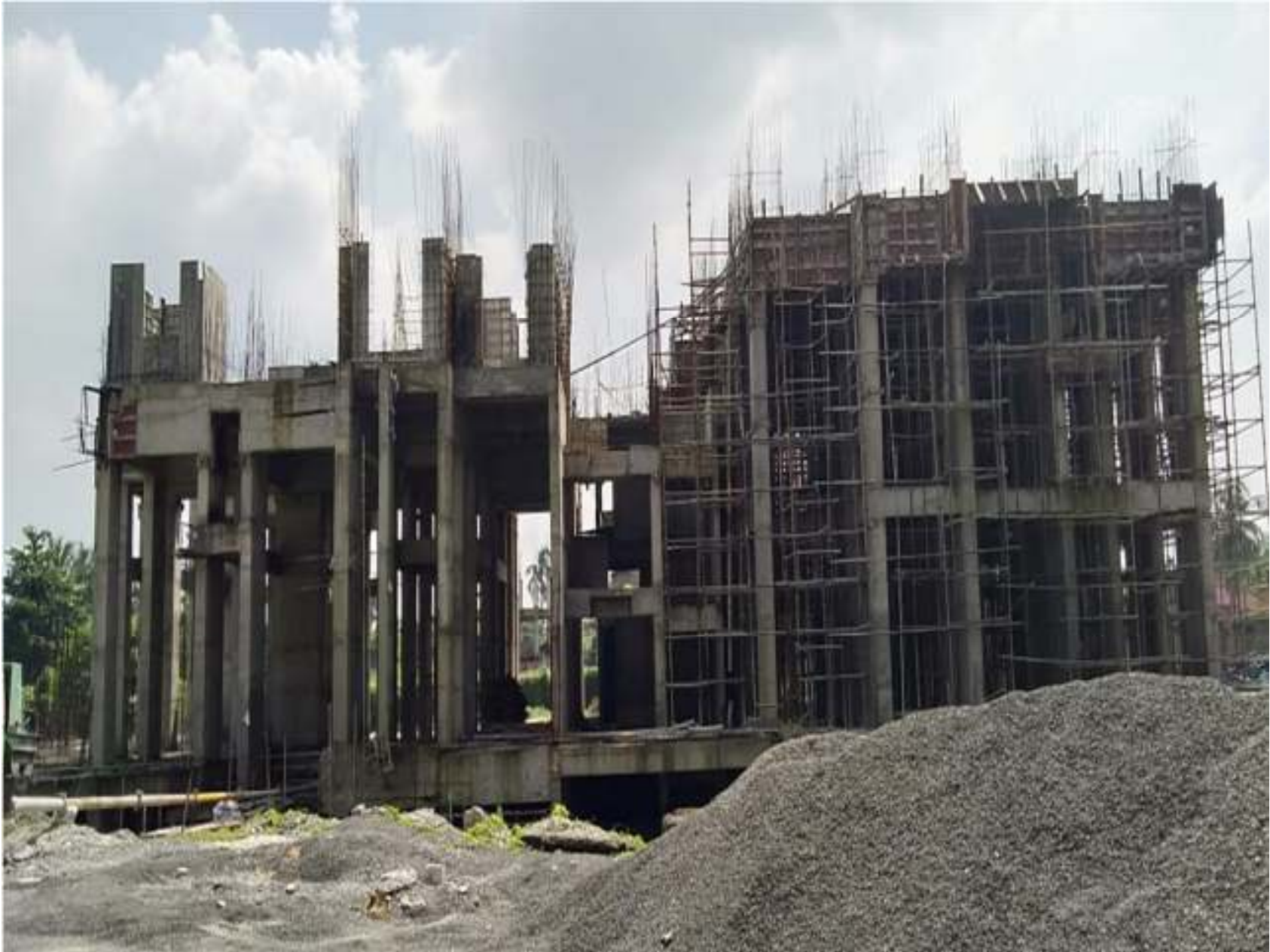
Block-7 (G) 50% of 3 rd Floor Slab casted.
