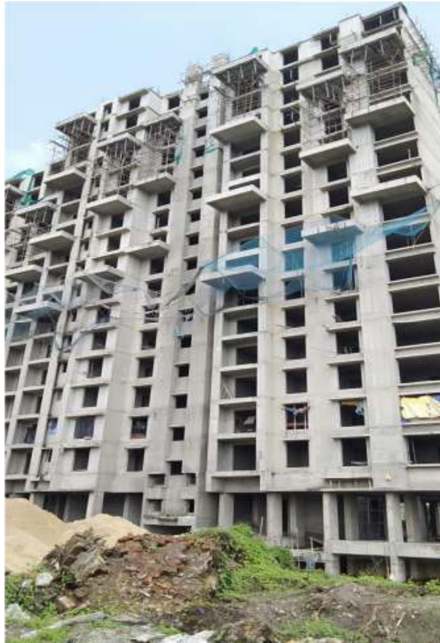
Block-4 (D) Terrace floor slab casted. Above Terrace wip.
